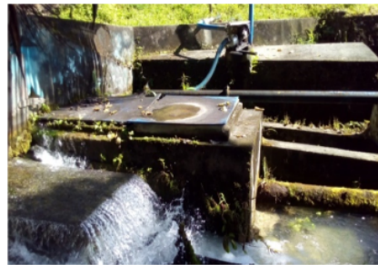
Figure 2. Mangkio water spring building.
