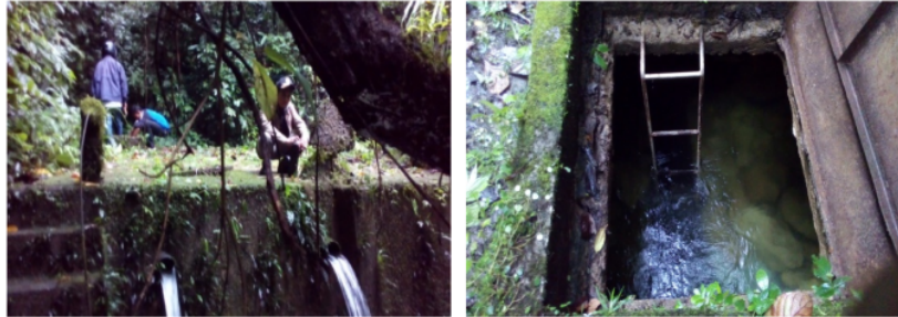
Figure 1. Keles water spring building.
