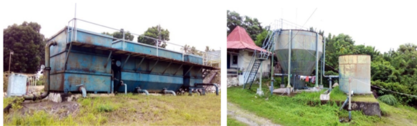
Figure 3. Water Treatment Plants (WTP) of Keles
